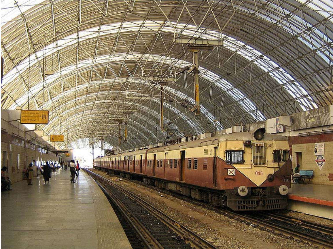
Dual gauge EMU on the Chennai MRTS in India
