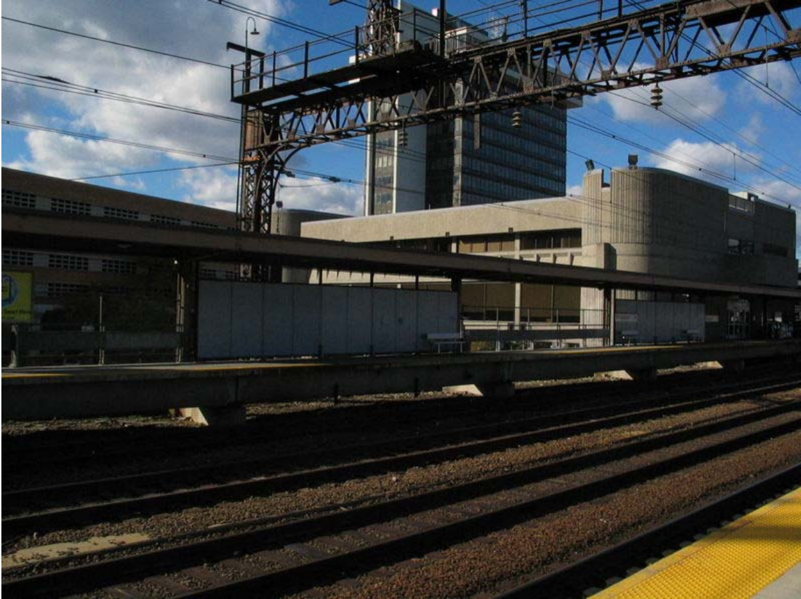
Overhead wire and catenary in Bridgeport, Connecticut, United States
