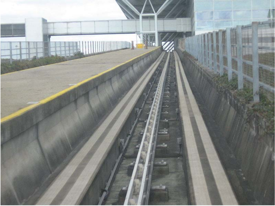
London Stansted Airport people mover central rail
