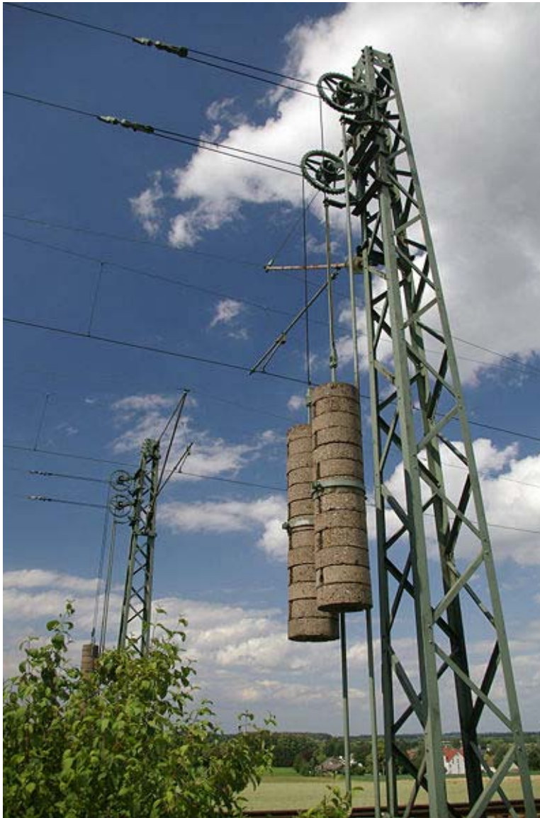
Line tensioning
