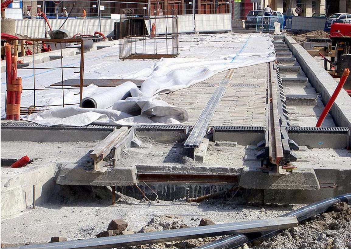
Track with APS under construction in Place Paul Doumer, Bordeaux
