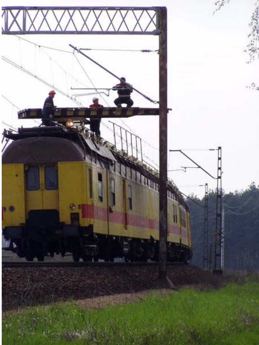
Linemen on a maintenance of way vehicle repairing overhead lines
