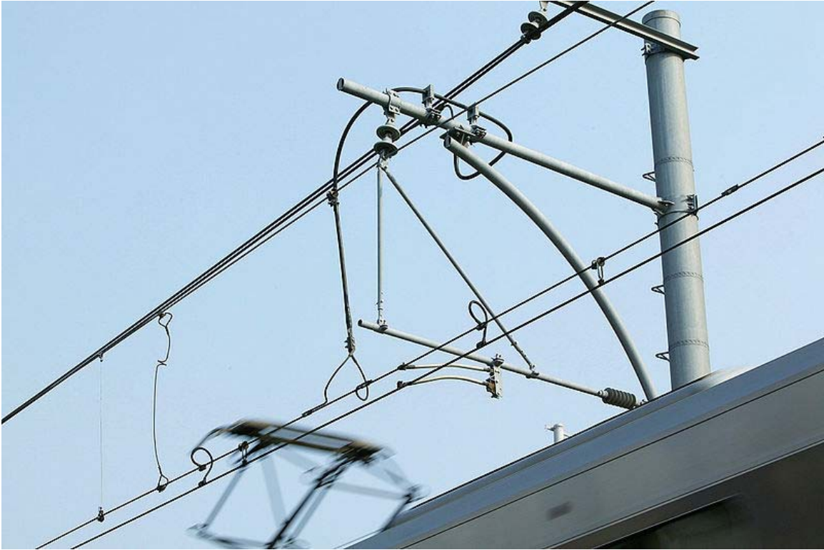
Compound catenary equipment of JR West
